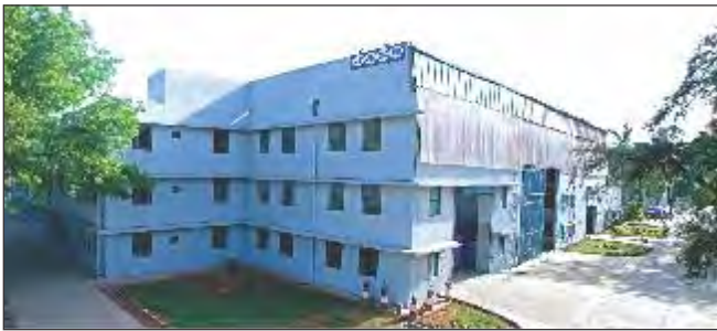
Sluice gate plant, Indore
