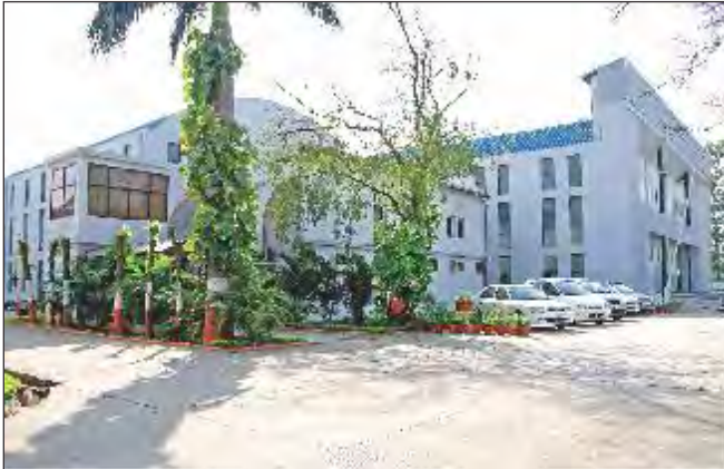
Knife gate valve plant, Indore
