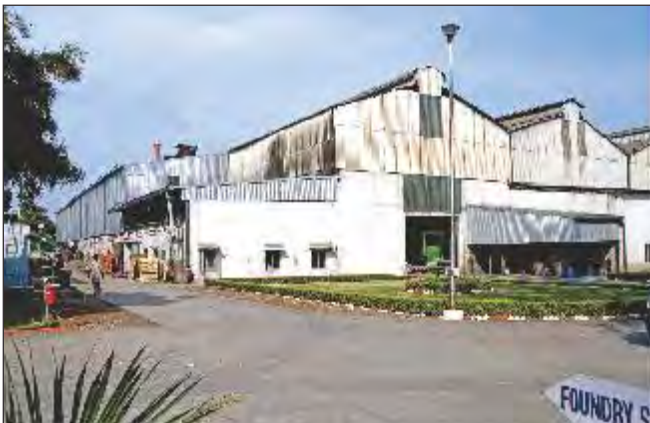
Cast iron foundry, Indore
