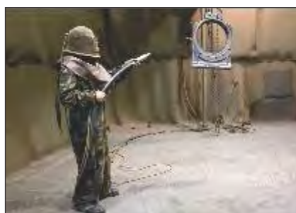
Shot blasting 6 x 6 x 24 m
